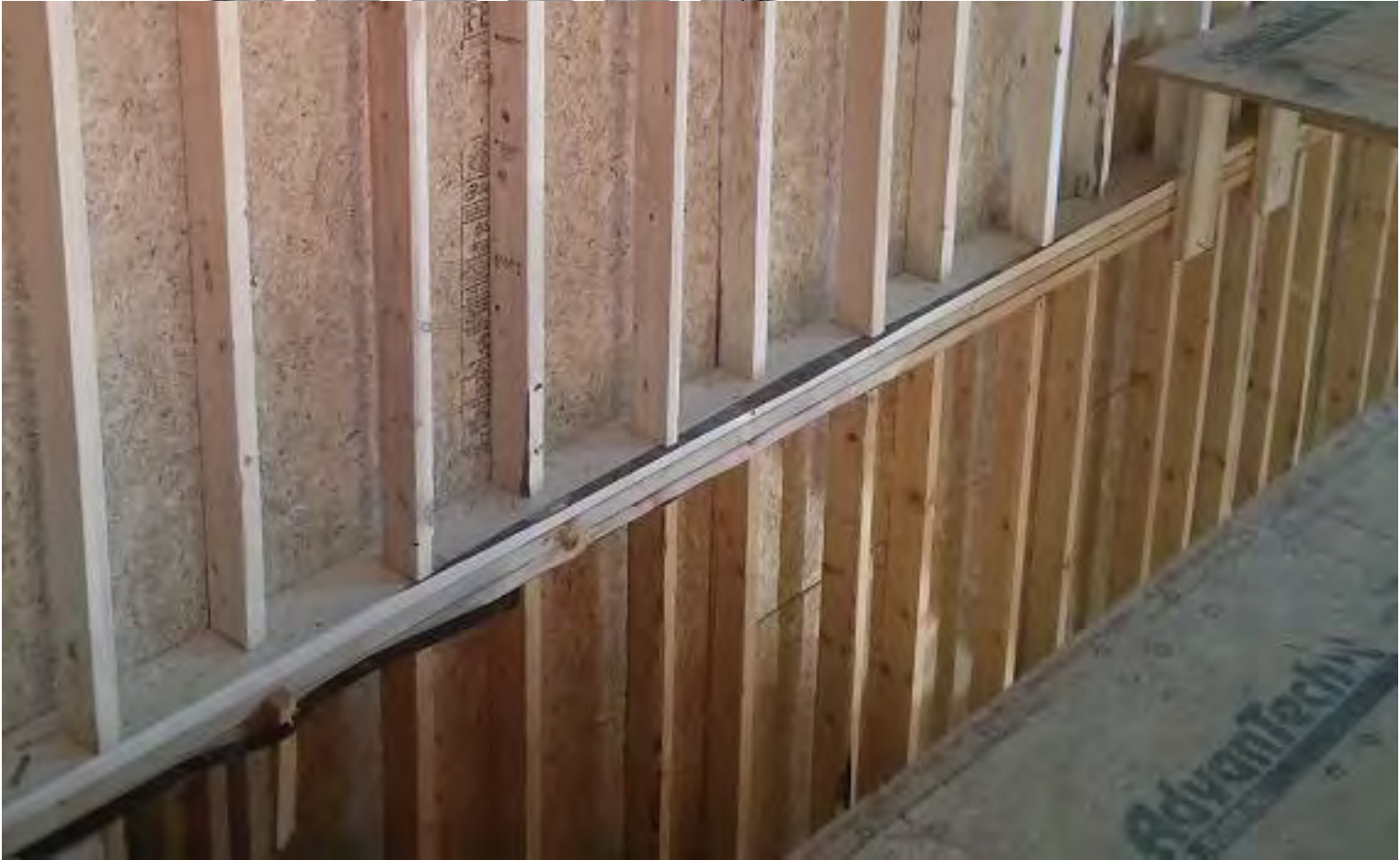
TYPICAL EXTERIOR FRAME WALL CONSTRUCTION
